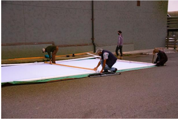
Drive-in screen assembly
