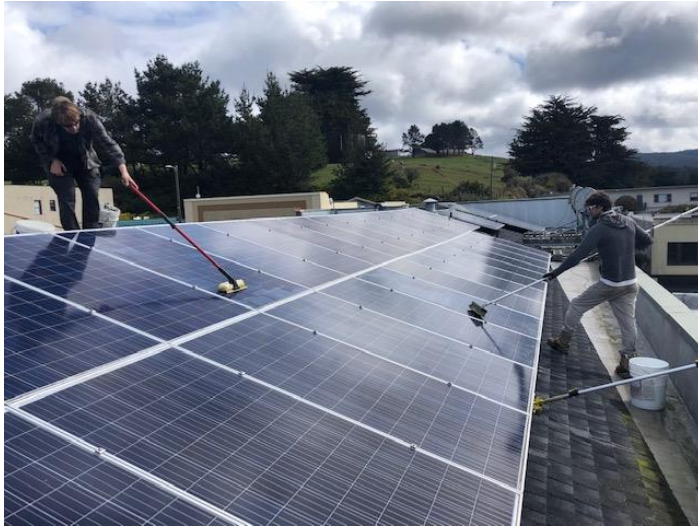
Spring cleaning of the solar panels
